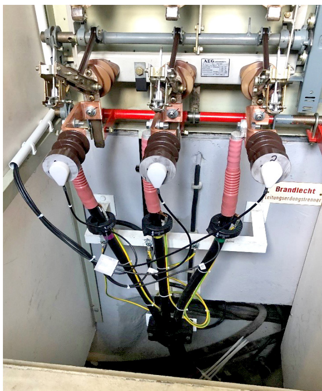
Retrofitted current and voltage sensors for load flow detection for each outgoing circuit.
